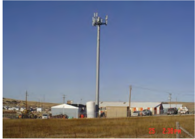
Looking from the flagpole location toward the monopole, this view looks 500 feet across separately owned vacant property that was not available for a wireless tower site lease. The author supplied this photo to the city council.
